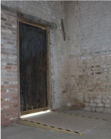
Access Ramp in East Barn
