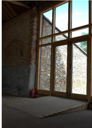
Access Ramp in Main Barn
