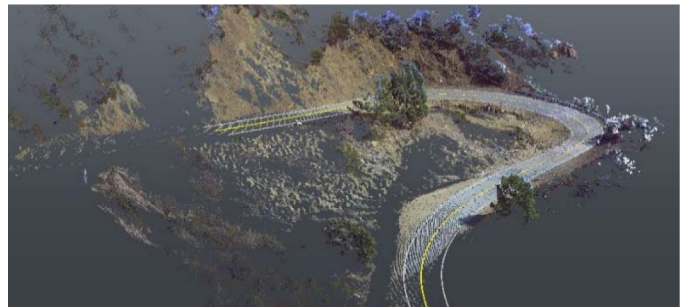
Figure 5. Survey and Scan Data of Edwards Corner Combined
