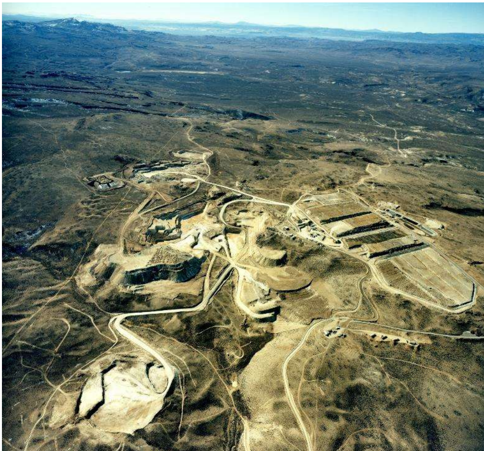
Figure 9: Aerial photo of the Hog Ranch Operation in 1989. View is looking south.
