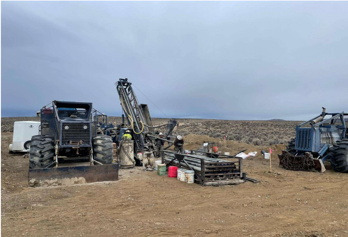
Figure 3: Drilling on the first drill hole at Airport.
