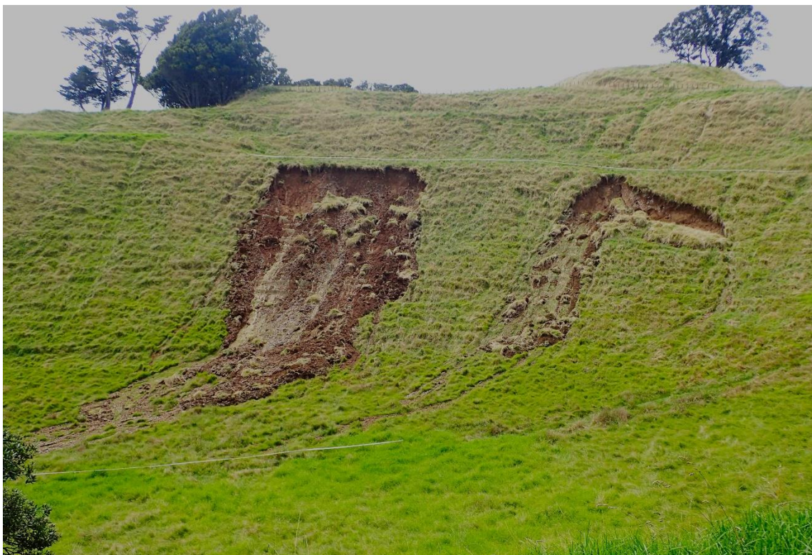
Fig. 3. The two largest slips (3-5) in the southwestern breached crater. Note how slip 3 (right) has started slipping at the top, just below the edge of the terrace above.
