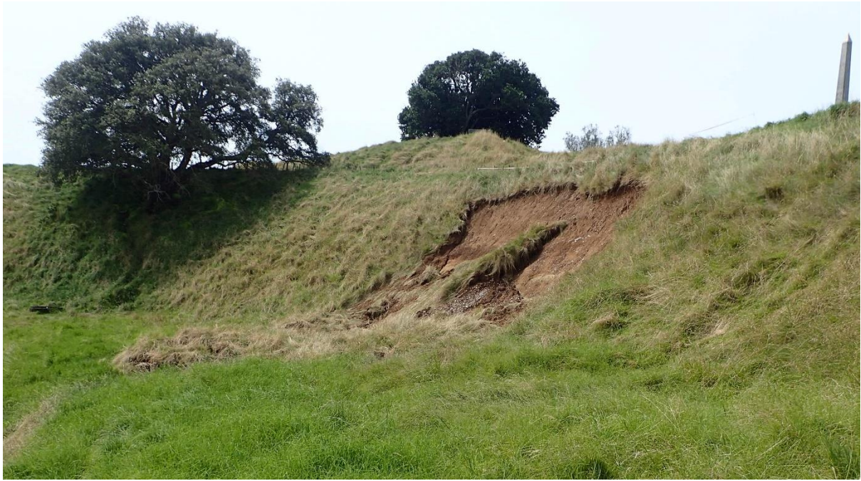
Fig. 6. Slip 1, in the southwest crater wall is an example of the kind of slips that have occurred on Maungakiekie, with failure of the rise between two terraces and only the upper 0.5-1 m of regolith failing and flowing down the slope with its toe extending across the lower terrace.
