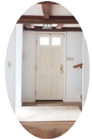
Existing Front Door
