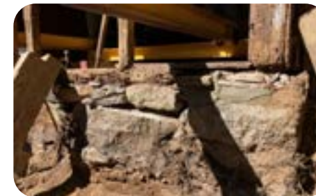
Dislocated foundation stones, which caused part of the house to sink and created a shelf that trapped water inside.
