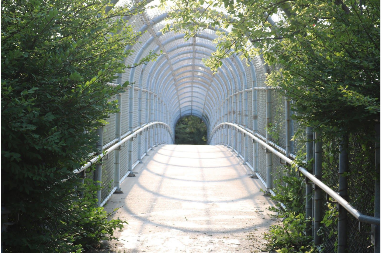
The Pratt Street Bridge
