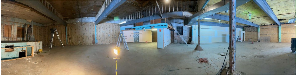
Construction underway on Culxr House's skatepark expansion.
