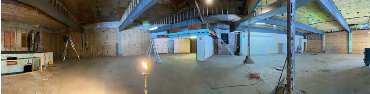
Construction underway on Culxr House's skatepark expansion.
