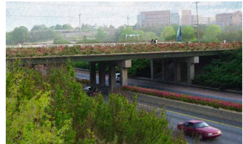
Until the bridges in this location get reconstructed, the existing ones can be enhanced with planters or green screens that extend the idea of park across the highway.
