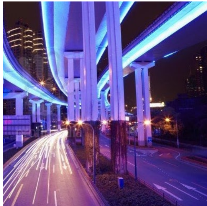
Utilize dramatic lighting for the undersides of the bridges and medians to create a "Corridor of Light."
