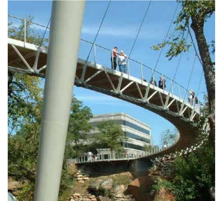
Liberty Bridge, Greenville, South Carolina
