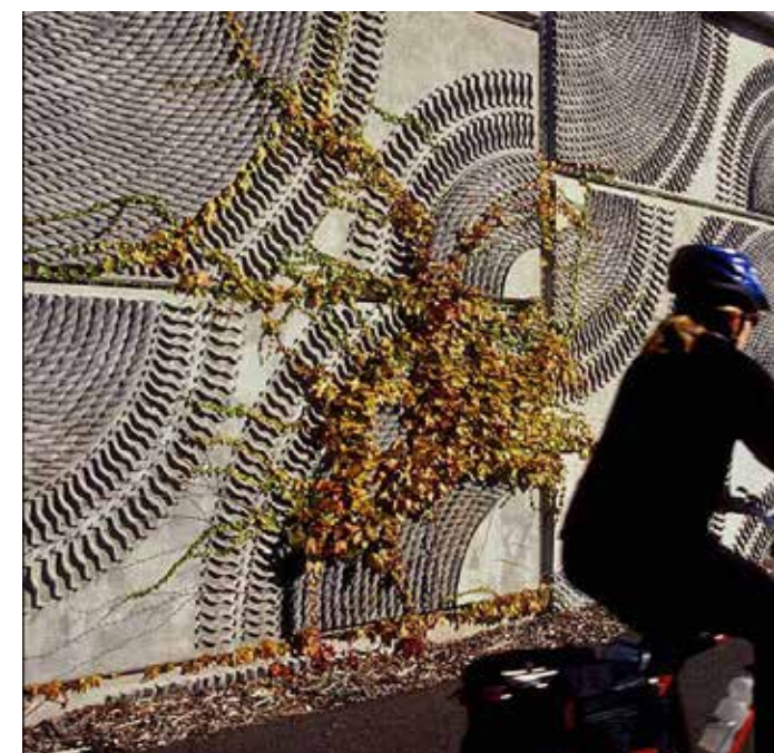
Artful Retaining Wall
