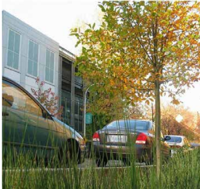
Within future street cross sections, consideration shall be given to providing water management landscapes along the edges of pavement.
