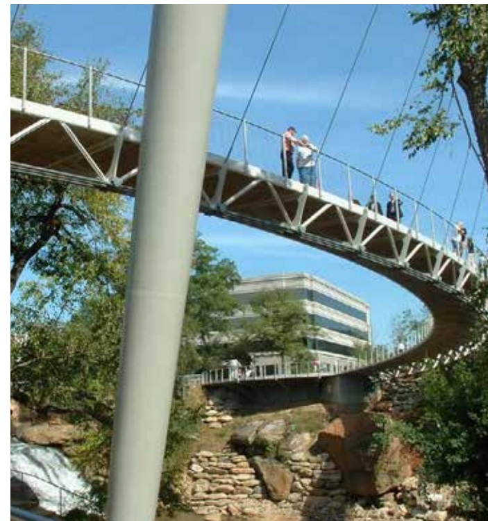
Integrate art into the design of structures such as the Linerty Bridge in Greenville, SC.
