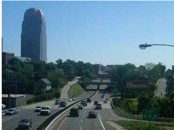
① The aesthetic experience of the Corridors would be enhanced with a cohesive design idea that creates consistency in the bridge forms and establishes a treatment for the center median that links the Corridor together.
