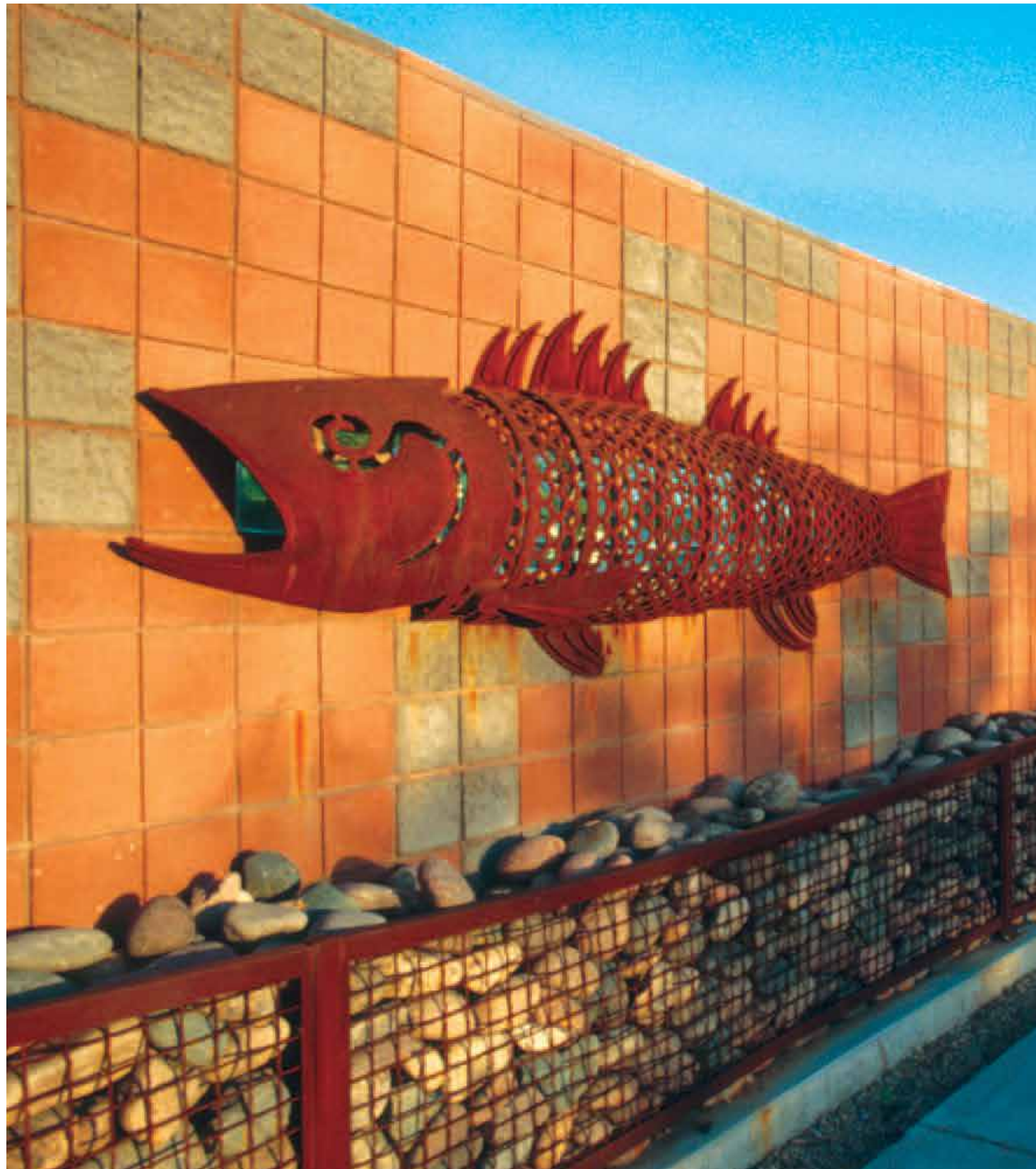
Different materials and art integrated into retaining wall
