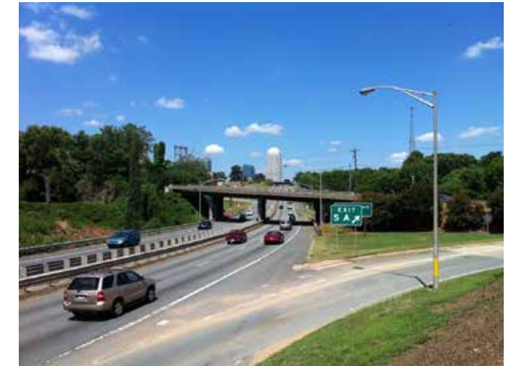
⑫ The view looking east at the Peter's Creek Parkway interchange with Downtown in the background.
