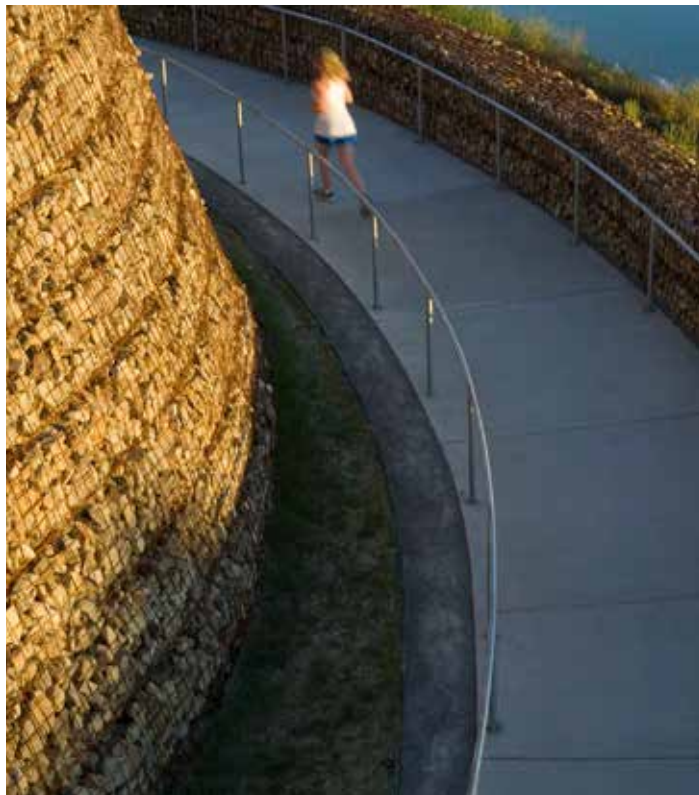
Gabion walls with pedestrian trail
