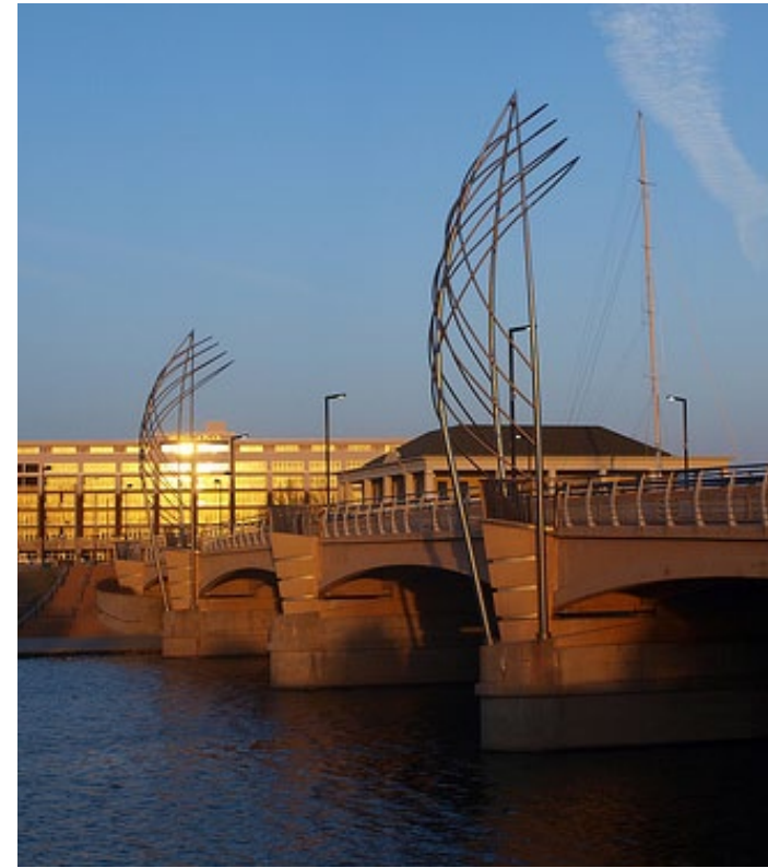
Vertical metal sculptural pieces on center pilaster like by Viki Scuri
