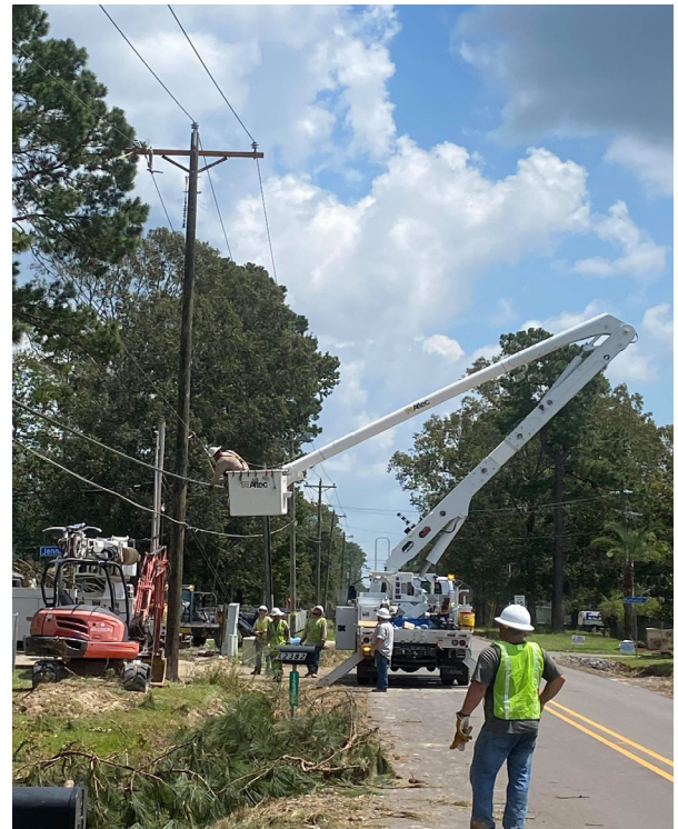
Right: Crew members in a bucket truck placing wire and equipment on a pole.
