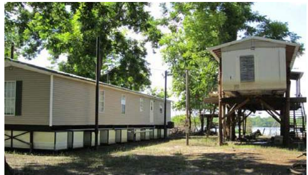
Figure 8. An amphibious home and one with PSE in Old River Landing, Louisiana, after flooding in spring 2011; note waterline on elevated house on right (photo by E C English)
