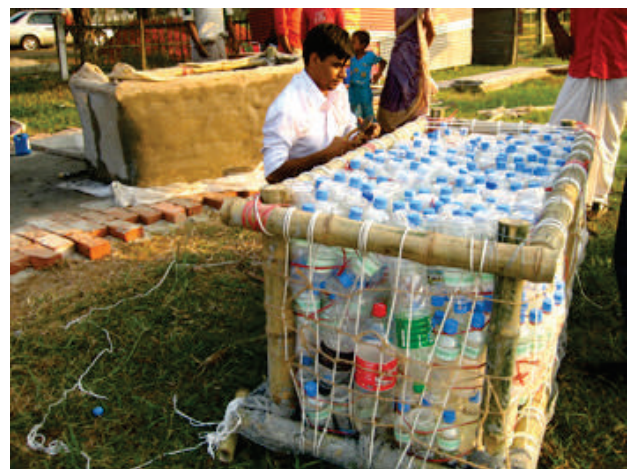
Figure 13. LIFT House buoyancy blocks using recapped plastic bottles (photo courtesy of Prithula Prosun)
