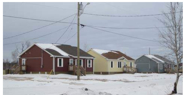
Figure 20. Modular housing near Pinaymootang, Manitoba (photo by E C English)
