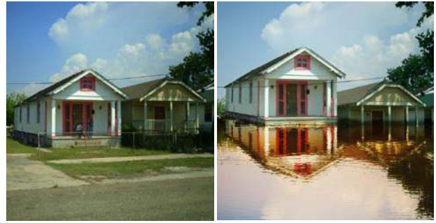
Figure 7. Amphibiation provides flood protection without significantly changing the building’s appearance (photo by E C English, renders by BFP)
