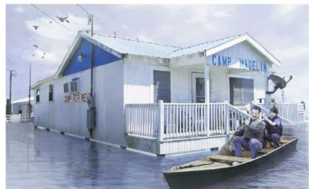
Figure 18. Camp Madelyn, Leeville, Louisiana, current condition and after amphibious retrofit (photo by E C English, render by BFP)
