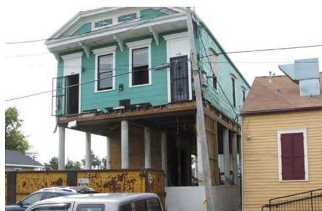
Figure 6. In New Orleans, permanent static elevation disrupts a neighborhood’s coherence and changes its character (photo by E C English)
