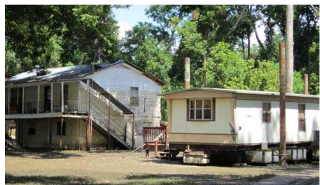
Figure 5. A static home (left) and an amphibious home (right) in Old River Landing, Louisiana; note waterline on static house marking depth of flooding (photo by E C English)
