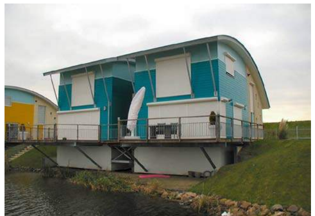
Figure 2. Amphibious housing in Maasbommel by Dura Vermeer and Factor Architecten (photo by Hans van Beek)
