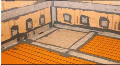
**14** Use Schlüter®-KERDI-COLL-L to create tightly sealed wall connections with Schlüter®-KERDI-KEBA sealing band.
