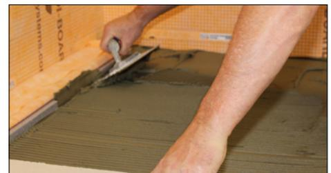
**6** Apply a bed of tile adhesive to the surface of the dry screed, ensuring the front edge of the drainage channel has adhesive underneath it.
