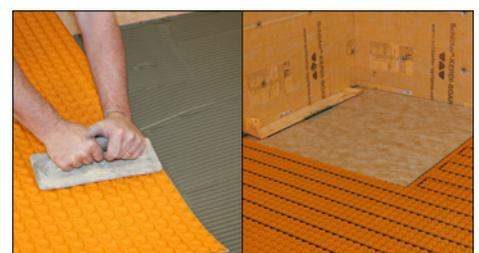
**9** If Schlüter®-DITRA 25 uncoupling membrane, or Schlüter®-DITRA-HEAT-E /-DUO underfloor heating is being used apply a bed of adhesive to the floor substrate and adhere the uncoupling membrane.
