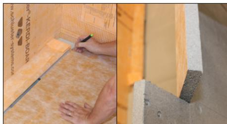
**5** Using a utility knife and the pre-printed markings on the back measure and cut out the sloped tray Schlüter®-KERDI-SHOWER to accommodate the drainage channel.
