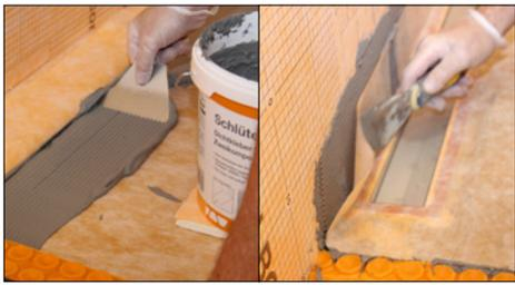
**10** Adhere the Schlüter®-KERDI collar, using the sealing adhesive Schlüter®-KERDI-COLL-L (see Product Data Sheet 8.4), to the adjoining waterproofing assembly with a 3 x 3 mm or 4 x 4 mm notched trowel and comb provided. Completely embed the Schlüter®-KERDI collar in this assembly, observing the curing times of all materials.
