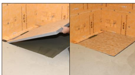
**8** Carefully place the Schlüter®-KERDI-SHOWER preformed shower board on top of the adhesive bed, sliding the tray under the flange of the drainage channel. Care should be taken to ensure the channel is not lifted.
