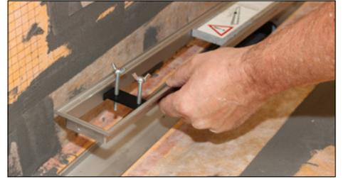
**15** Insert the frame with the spacer strip. If the 30mm high frame is being used (only suitable for use with a central outlet position) carefully adjust the grate support feet around the trap so the trap can be removed for cleaning.
