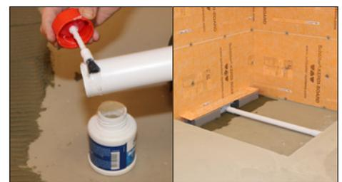
**3** Connect the drain outlet to the building drainage system, ensuring an appropriate fall to the waste pipe. Check for leaks.
