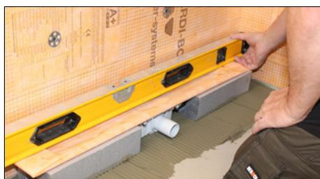
**2** Using a spirit level adjust the drain until it is level along its length and across its width. If necessary, apply spots of tile adhesive for height adjustment. Remember that for wall installation, the thickness of the tile or stone covering the wall must be taken into account. If necessary, use the polystyrene fill strip provided.
