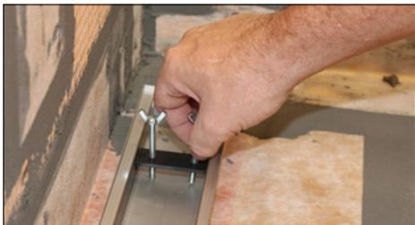
**16** Use the supplied height-adjustment aid to adjust the frame to the thickness of the tile covering.
