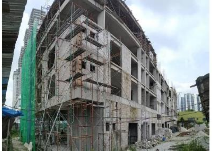
Figure 9: Construction site of commercial property project in Sentul
