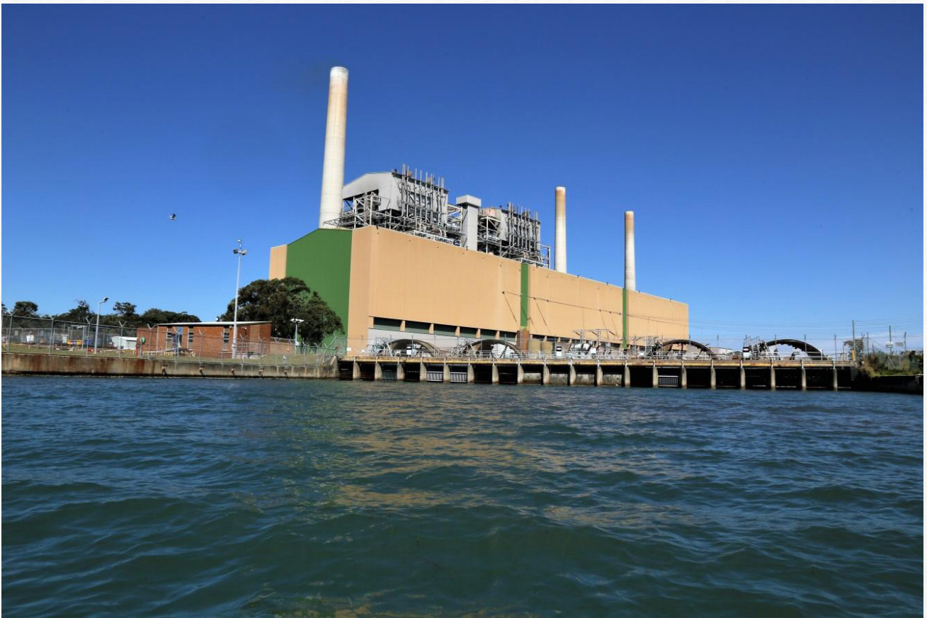
Figure 3 Vales Point power station cooling water intake Chain Valley Bay
