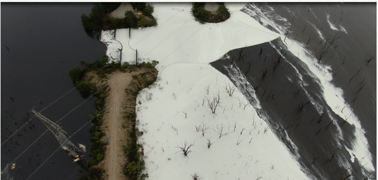
Figure 32: Settling ponds of Vales Point Ash Dam before release to Wyee Dam.
