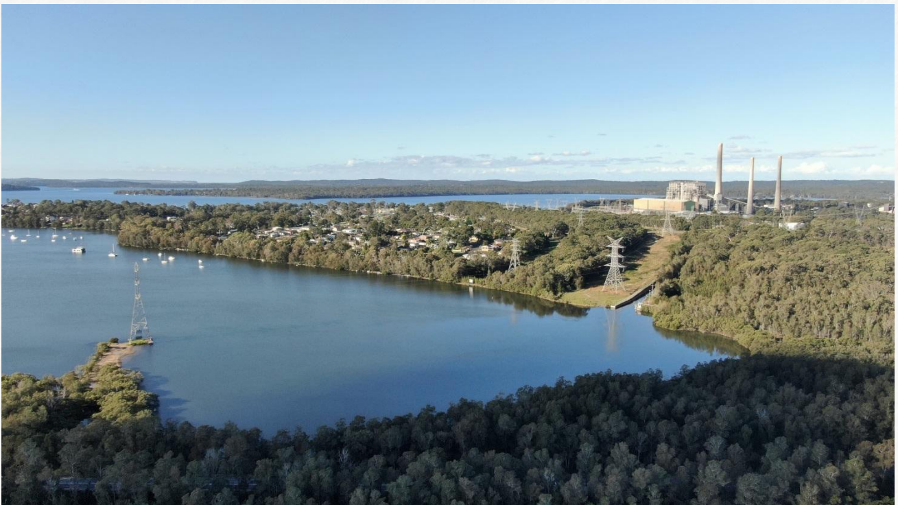
Figure 6: Vales Point hot water outlet and Wyee Bay
