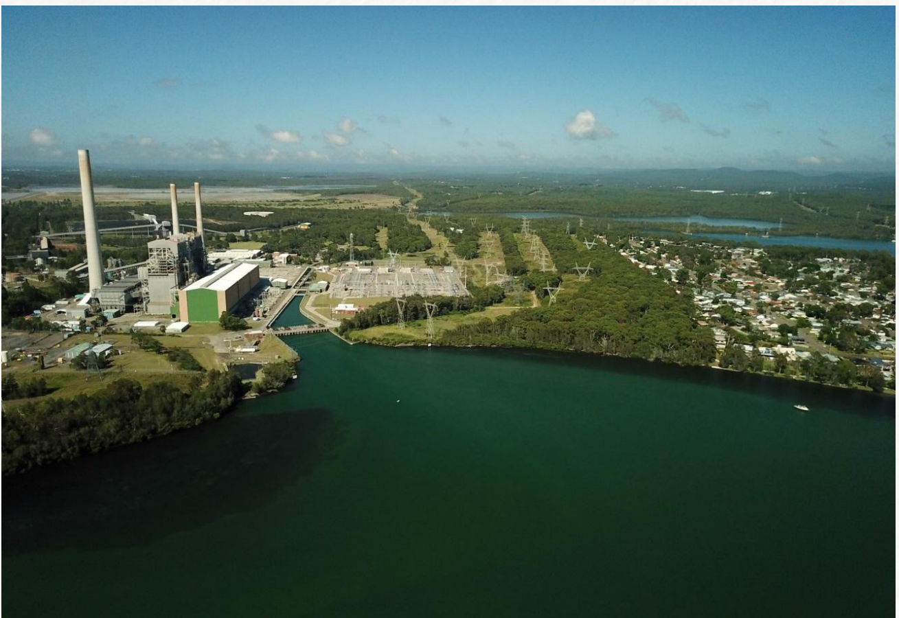
Figure 4: Vales Point intake
