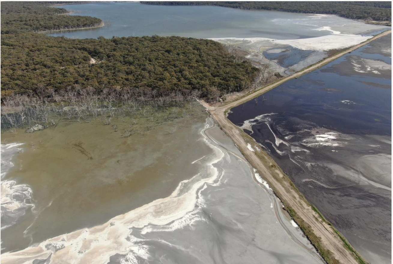
Figure 34: Excessive water collecting in Vales Point Ash Dam
