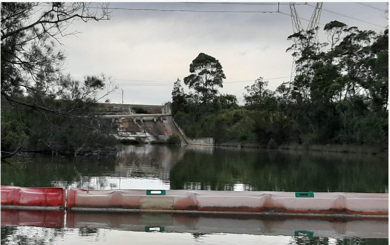
Figure 30: Original ash dam overflow into Mannering Bay
