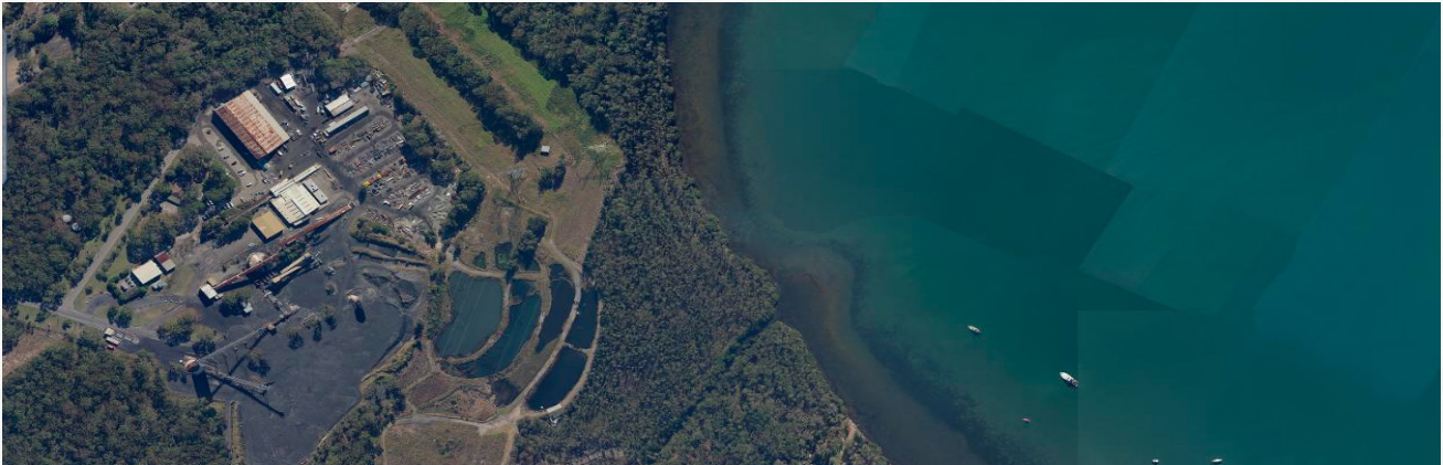
Figure 35: CVC pit mouth, discharge settlement ponds, and Swindles Creek mine discharge.
