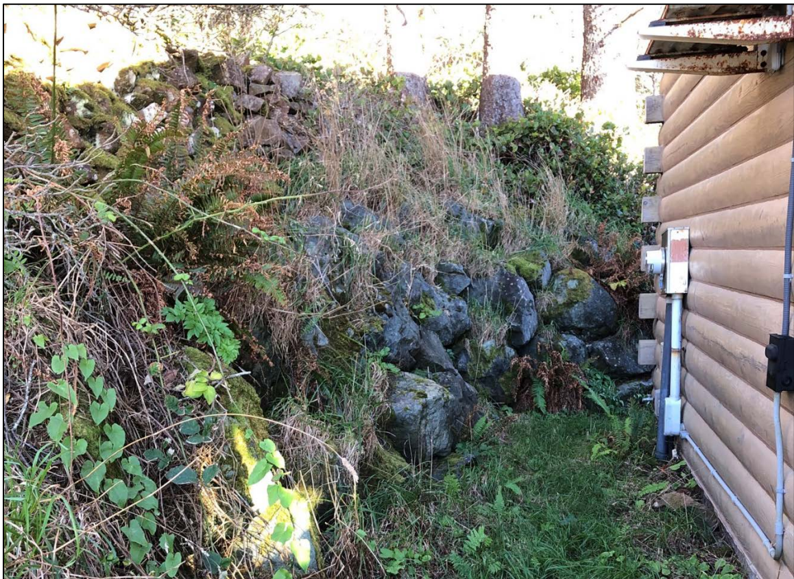
Photo 4: Rockery wall located north of the existing residence, facing east.
