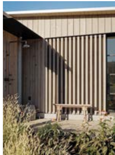
Two cement cores stand either side of the main living area. One forms the chimney and the second embraces the kitchen cabinetry. The kitchen itself was envisioned as a solid block of wood in which the counter was carved out to add to the crisp aesthetic and clean lines of the architecture
