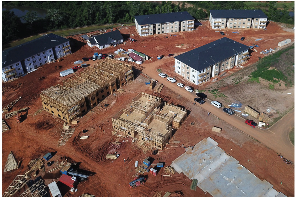
Camellia Commons of Enterprise, AL - New construction of 176 apartments
