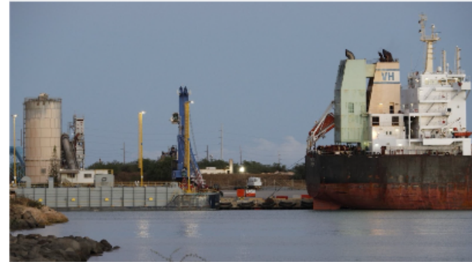
The last barge of coal arrives to O'ahu to fuel the coal plant, signaling the end of the island's dirtiest energy source. (Photo Credit: Hawai'i State Energy Office)
