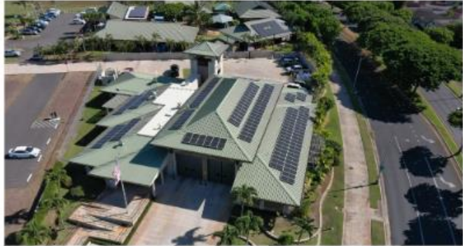
New 56 kilowatt solar photovoltaic system on the roof of the 'Ewa Beach Fire Station. (Photo Credit: Department of Design and Construction)
