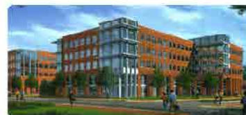
Building with appropriate orientation to street
