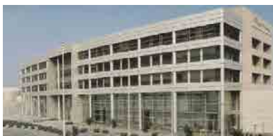
Office building with extensive window daylighting
