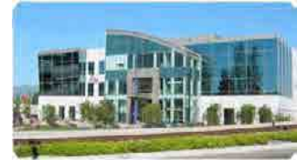
Enhanced entry and corner features
