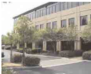
Contrasting color and congruent roof theme; note defined pedestrian path
