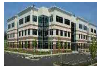
Differentiation of building with, colors, materials, and building plane changes
