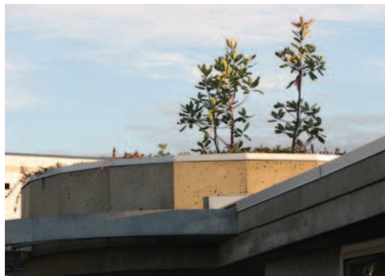
Top photo: Green roof on garden shed, Michigan Street Community Garden. Bottom photo: Green roof on Burnside-Gorge Community Centre. PHOTOS: CAROLYN MASSON
