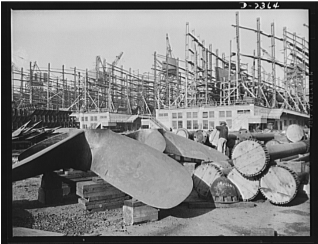
Image 6. Shipbuilding. “Liberty” ships. The propellers and shafting pieces are awaiting installation in the ships of the Liberty Fleet being built at a large Eastern shipyard. Source: United States Office Of War Information, Palmer, Alfred T, photographer, Baltimore United States Maryland, c. 1941.
