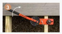
**LOCK-IN** Apply pressure by moving the handle towards the deck board. Do not overtighten as the boards can buckle.
