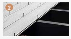
**REPEAT ALONG THE BOARD** Place a clip at every joist along the length of the board.
