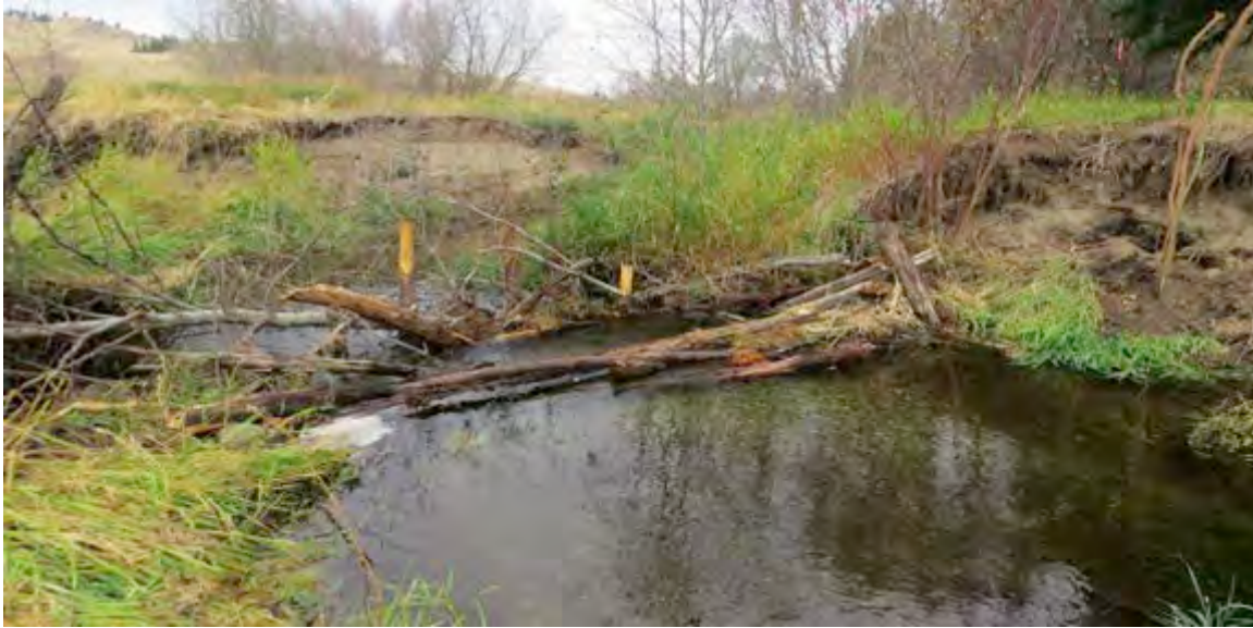
Figure 77: 12 days following installation of a BDA (same location as figure 81) and placement of LWD and other debris showing water pooling upstream
