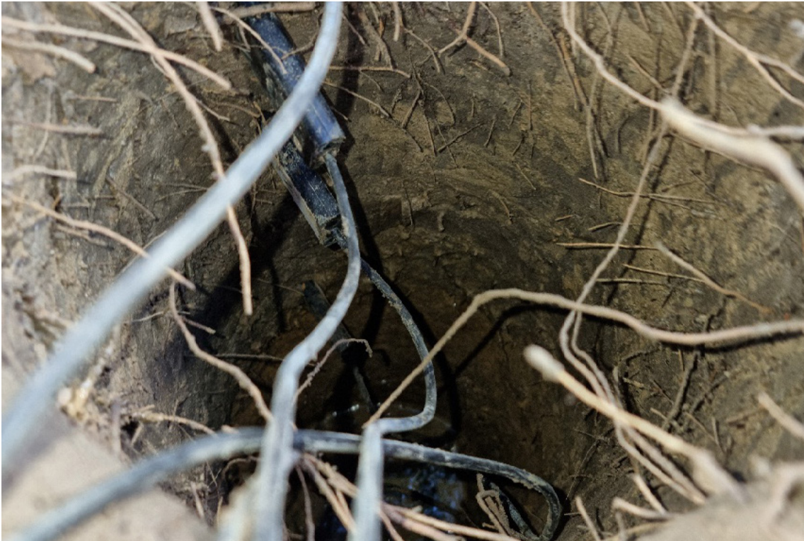
Figure 4. Soil moisture sensors installed horizontally into key depths within the rootzone. Sensor depths are 10cm, 20cm, 30cm, 50cm, 80cm.
