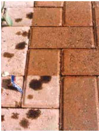
Figure 3. It is easier to remove oils stains from pavers that have been sealed.
