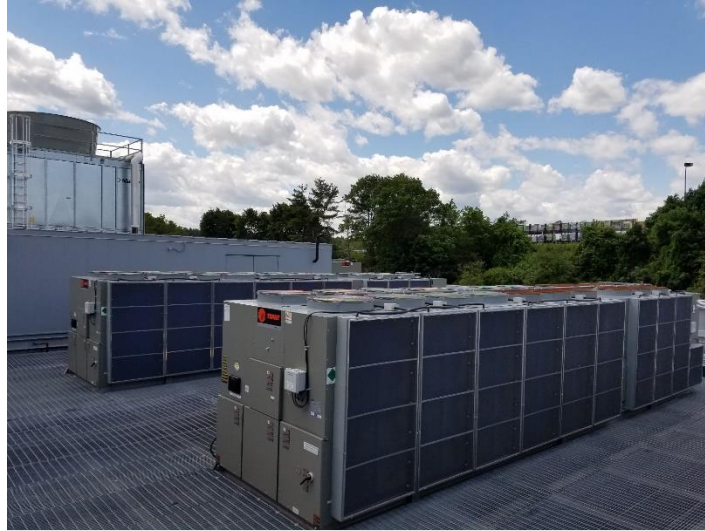
Figure 2: Peak+ installed on two air-cooled chillers.
