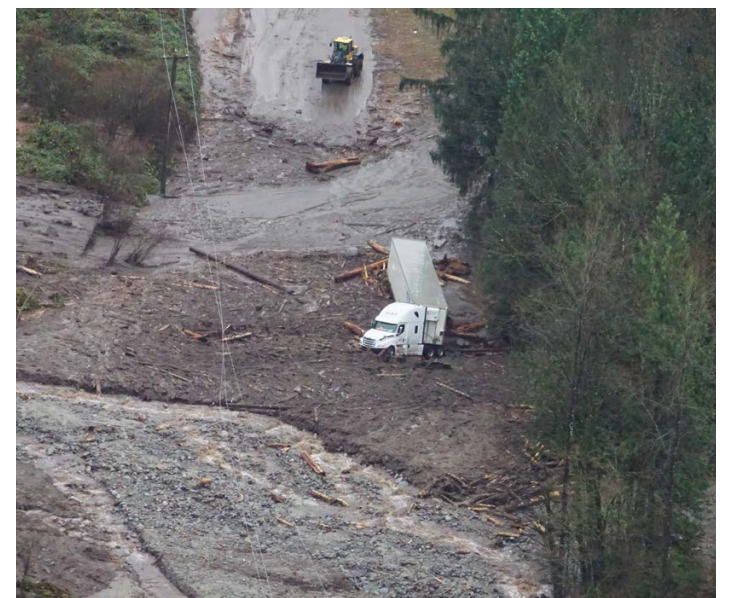
Figure 4. One of several debris flows that affected the Trans-Canada Highway and the CPR Railway, November 2019. This debris flow blocked both lanes of the highway and the railway line, engulfing a semi-trailer truck. Photos: Matthias Jackob
