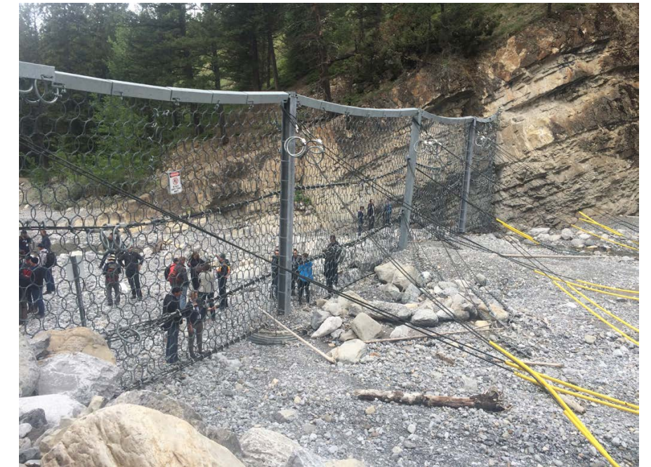
Figure 3. Temporary retention net installed on Cougar Creek upstream of Canmore. It is designed to slow and capture debris flows before they affect downstream infrastructure. A larger permanent structure is presently being built. Photo: Brent Ward, 2018
