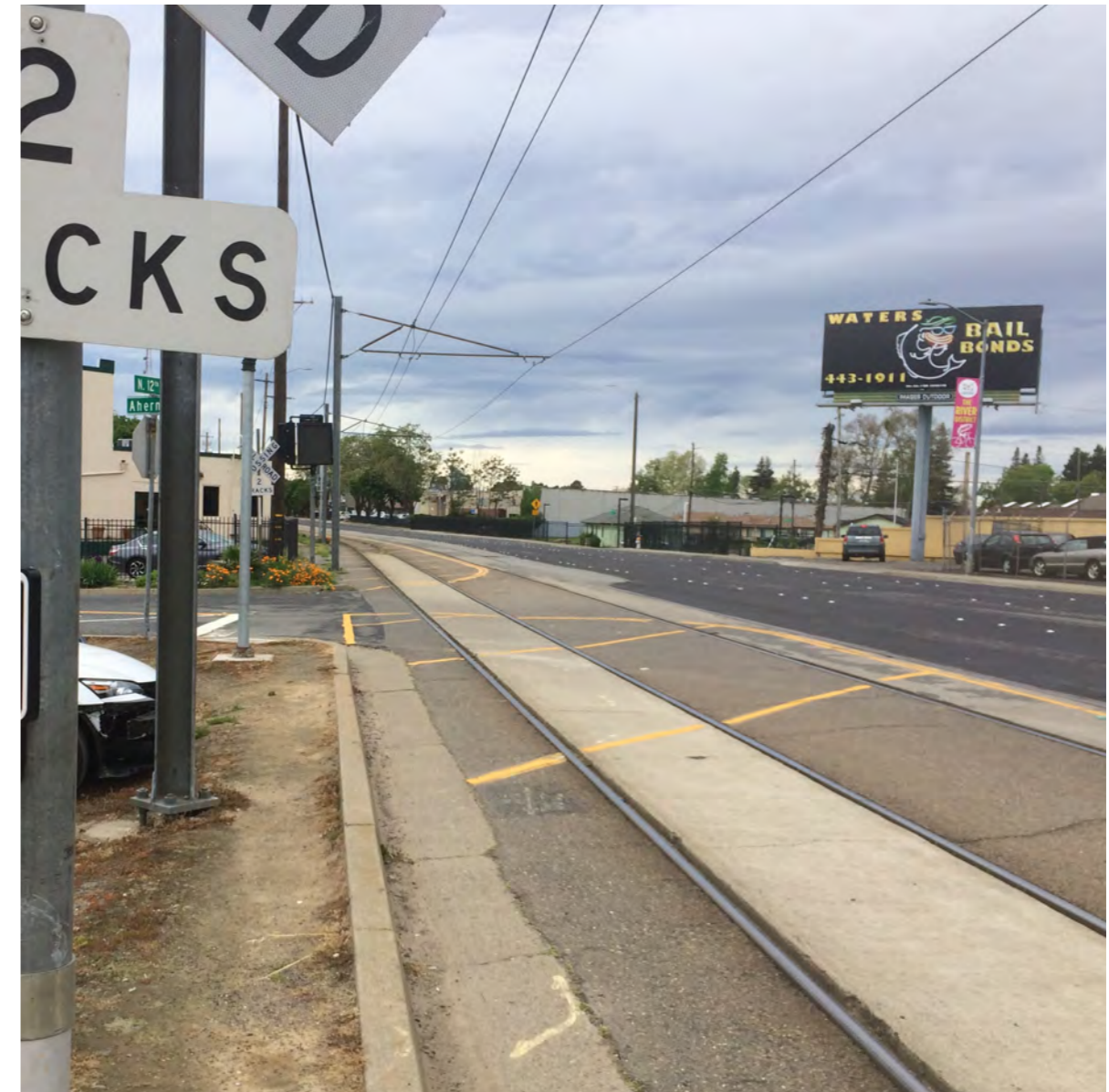
Looking down tracks at the end of the Dos Rios Station Site.
