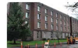
Building facing Jarrett St
