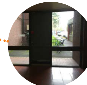
Existing East Lobby
