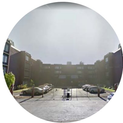
Existing Condition West Elevation
