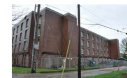
Building facing the Alley
