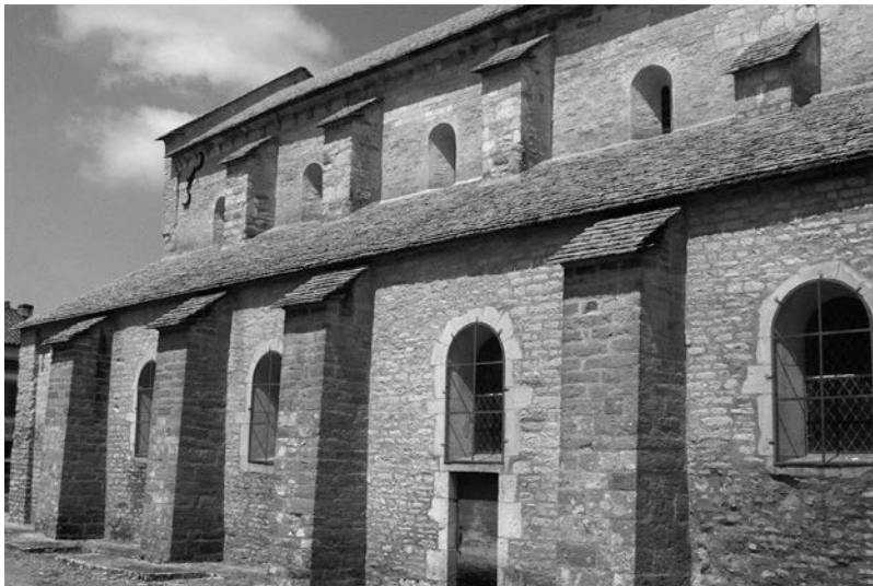
Figure 1. Buttresses treated architectonically to be incorporated into the body of the church, Saint-Martin, Chapaize, France.
