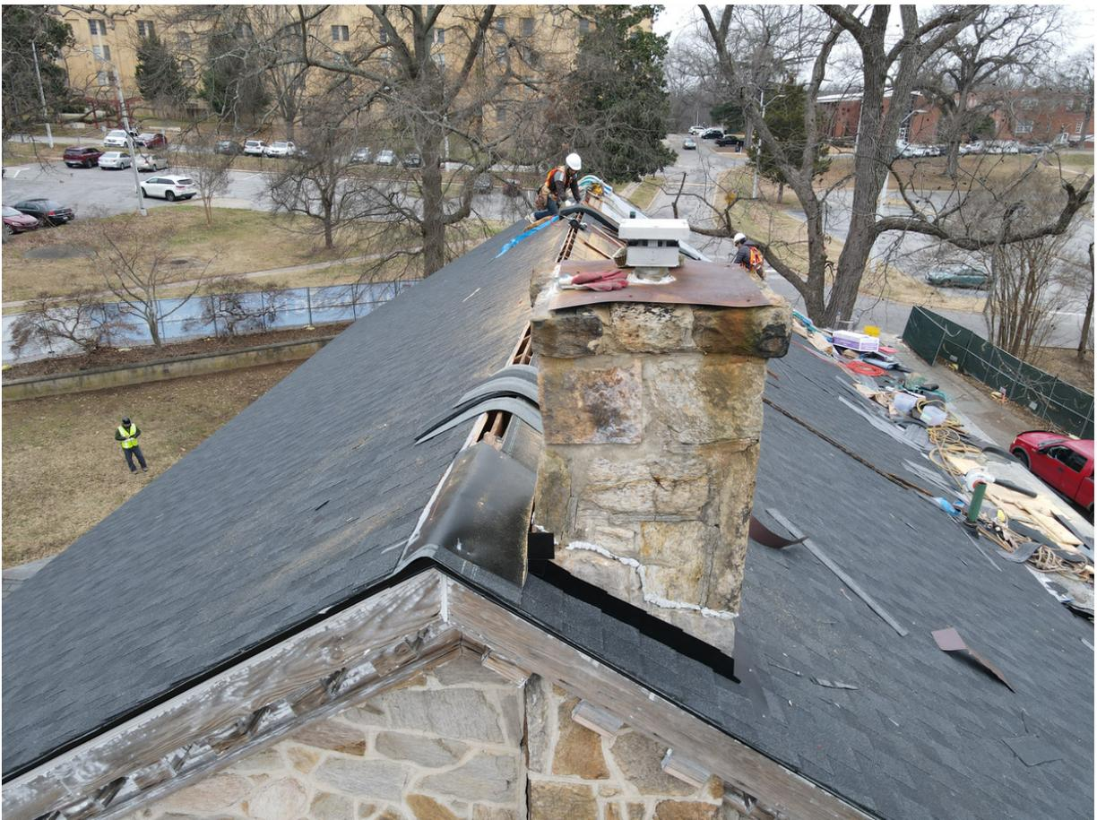
We have completed the reroofing of all buildings. The shingles were past the expected life span and were allowing water intrusion in some areas.
