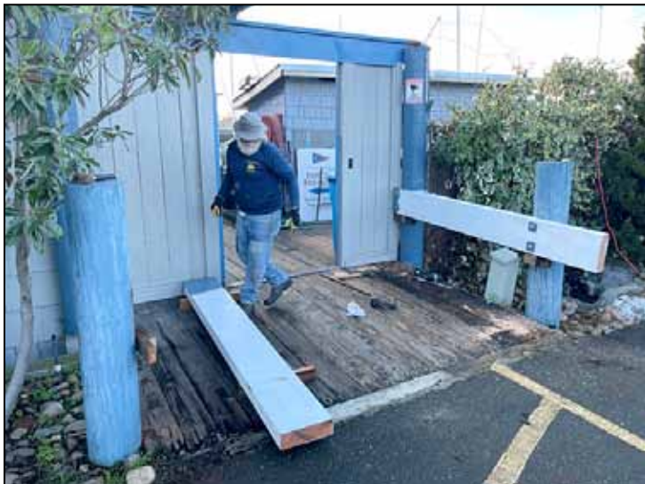
New railings by Jeff Ruszler. Photo courtesy Michael Read
