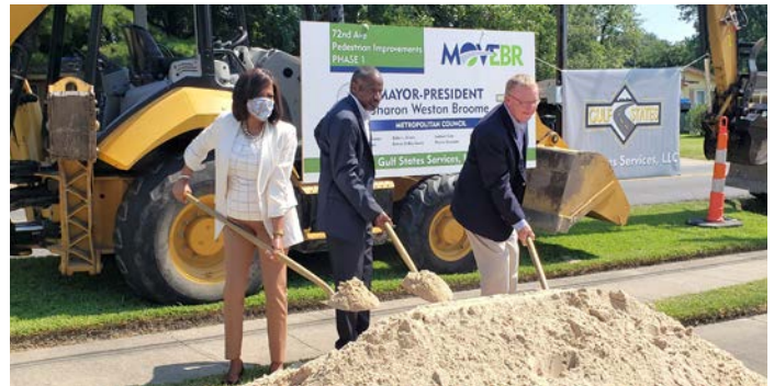
Groundbreaking of MOVEBR sidewalk construction on 72nd Ave. Source: move.brla.go
