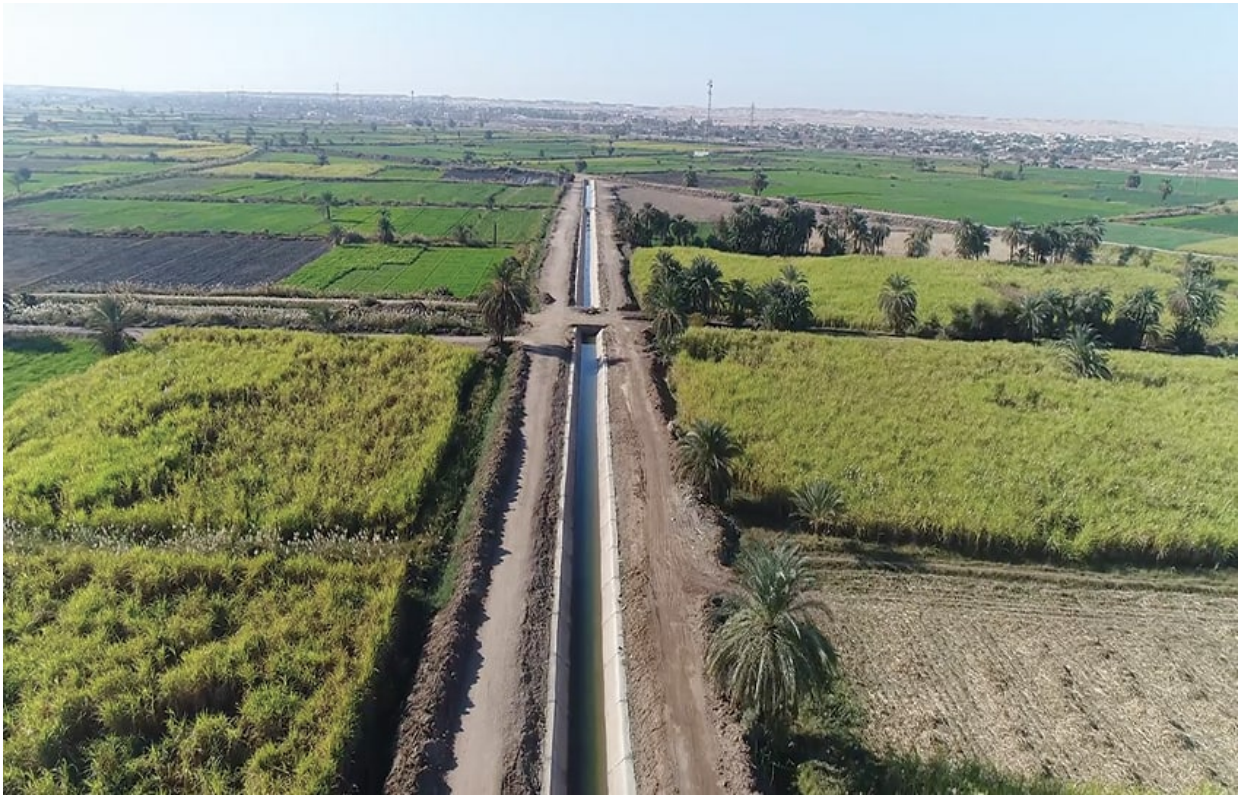
Lining canals to reduce water losses
