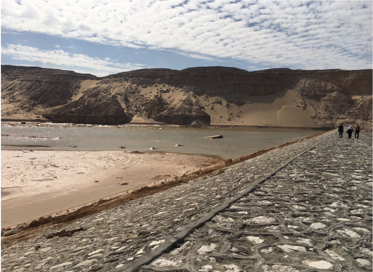
Flash flood protection
