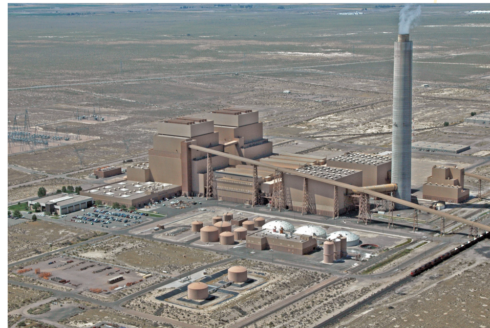
Intermountain Power Project, Courtesy of LADWP
