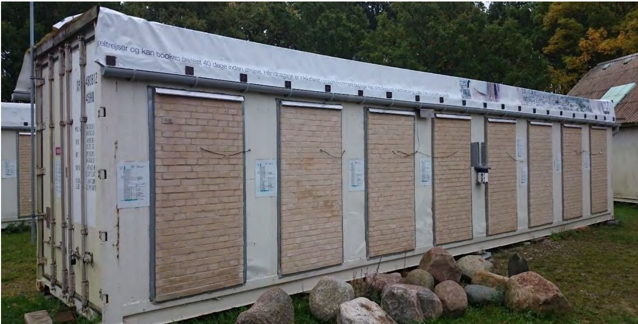
Fig. 50.: External view of the GI container.
