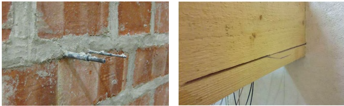
Fig. 14.: Inserted holes with test tubes in the bed joint of the masonry as seen from the cold side (left) and sawed cut in the joist end as seen from the war side (right).
