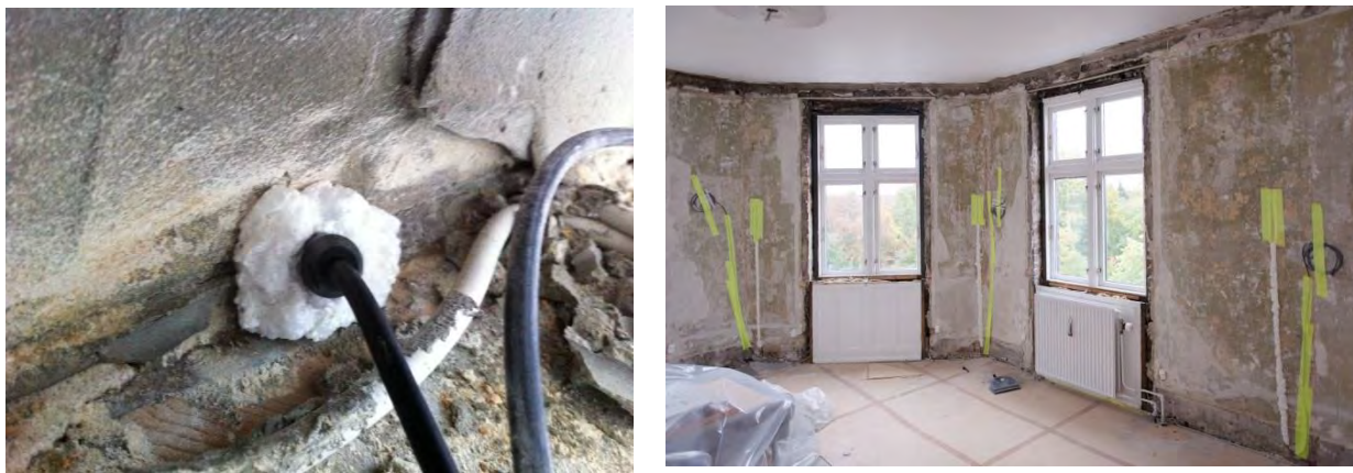
Figure 47: Placements of sensors behind beam-ends (left), drilled and sealed with foam, and in notches in the interior render (right), notches for the wire sealed with foam
