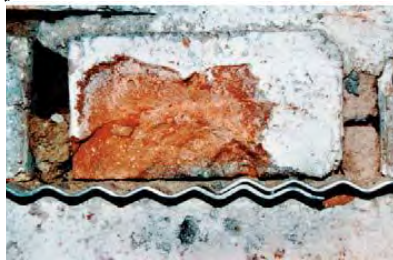
Figure 4–21: Examples of continuous moisture barriers (Source: Morten Hjørsløv Hansen (left and middle), (BYG-ERFA, 1997) (right)).
