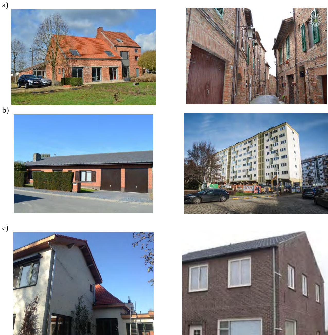
Figure 4–22: Driving rain load on a façade will in general be higher for a) a free standing building in an open region compared to terraced houses in the city, b) a high rise building compared to a low rise building and c) facades without physical protections due to overhangs etc.
