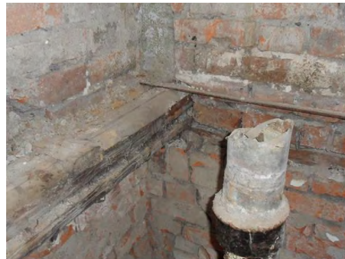
Figure 4-29: Possible damages as a result of a) an anchor or b) a damaged water pipe.
