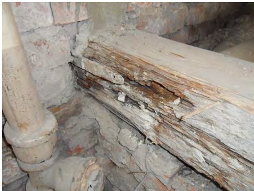
Figure 4-29: Possible damages as a result of a) an anchor or b) a damaged water pipe.
