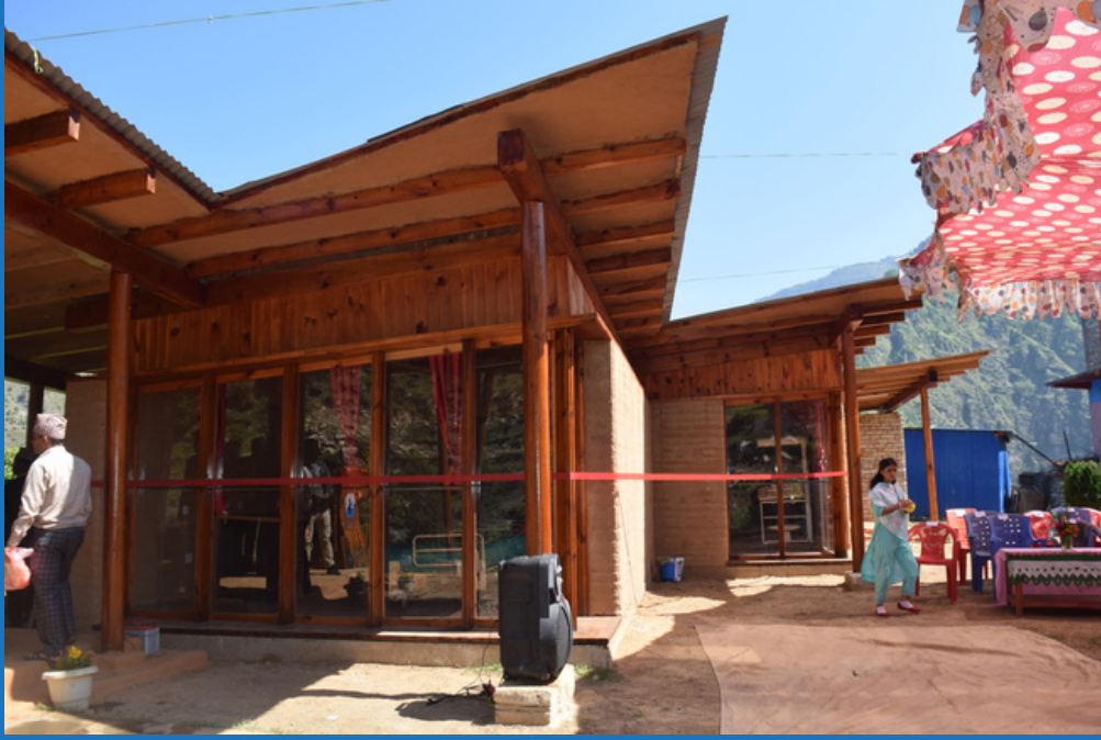
The completed Odanaku Birthing Center was completed in Fall 2021
