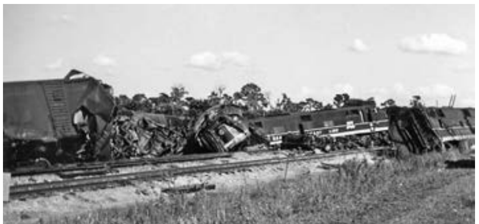
At right: These scenes look south and southeast and show the most heavily damaged cars and locomotives. Note the Seaboard 6050-series baggage-dormitory car and SAL box express car 742, the first two cars on the southbound train. The baggage-dorm suffered only light damage but No. 742 was a total loss. — Stan Jackowski photos
