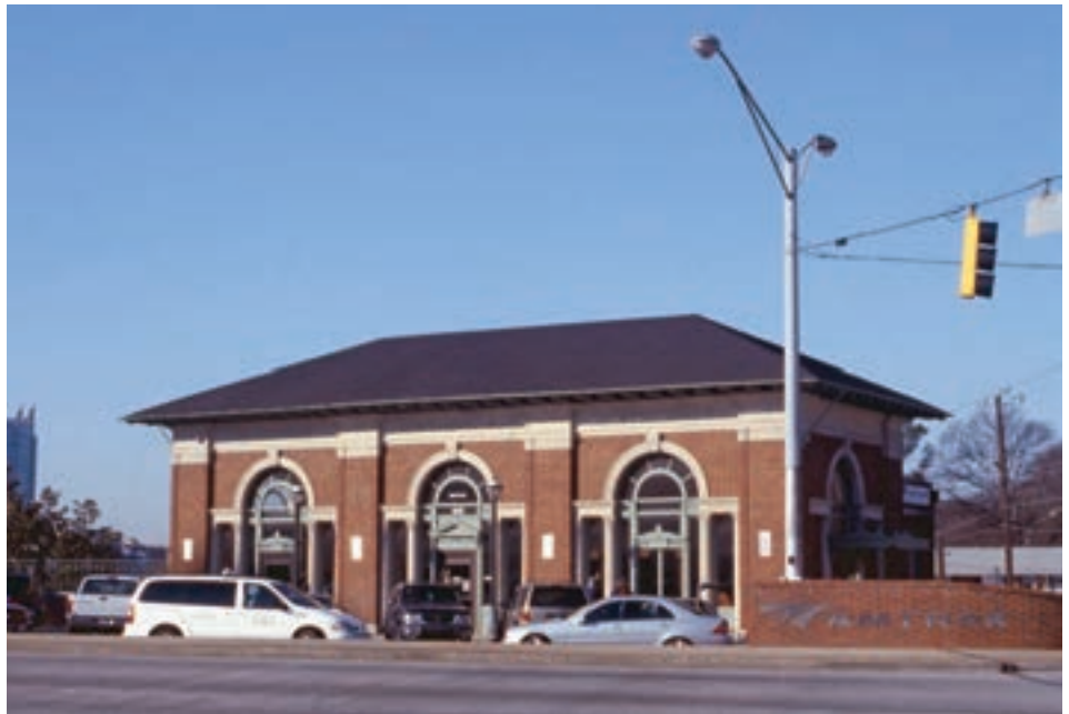
The ex-Southern Railway suburban Brookwood Station, shown here in March 2009, is the only surviving active passenger station in Atlanta. It is served by Amtrak's New York–New Orleans Crescent .
