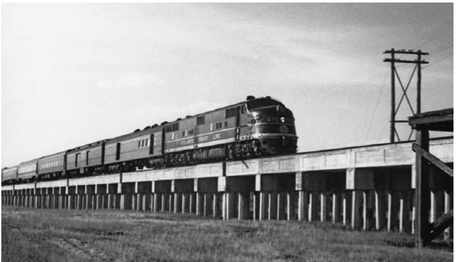
Above: Baggage-coach 666 was assigned to Atomic Energy Commission service between the Savannah River Plant near Augusta and Rocky Flats, Colo., carrying material to manufacture nuclear weapons. The car's interior was rebuilt to accommodate lead-lined containers and dormitory space for armed guards. This circa mid-1960s photo shows it in Chicago. — Jay Williams collection
