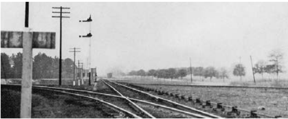
BX Tower operator F.W. Thomas was facing railroad south toward Gainesville on the Florida Southern Route, standing just south of BX Tower and the water tank, when he took this 1942 photo. The switch in the foreground, the only one controlled by the interlocking plant, is to the short connector (dog-leg), which curves around to the left to the long connector or north leg of the wye. The home signal for northbound Florida Southern trains can be seen just beyond the switch. All distant signals on all routes were fixed in the approach position; only the home signals were controlled by the interlocking plant. —F.W. Thomas photo, L.A. Bailey collection
