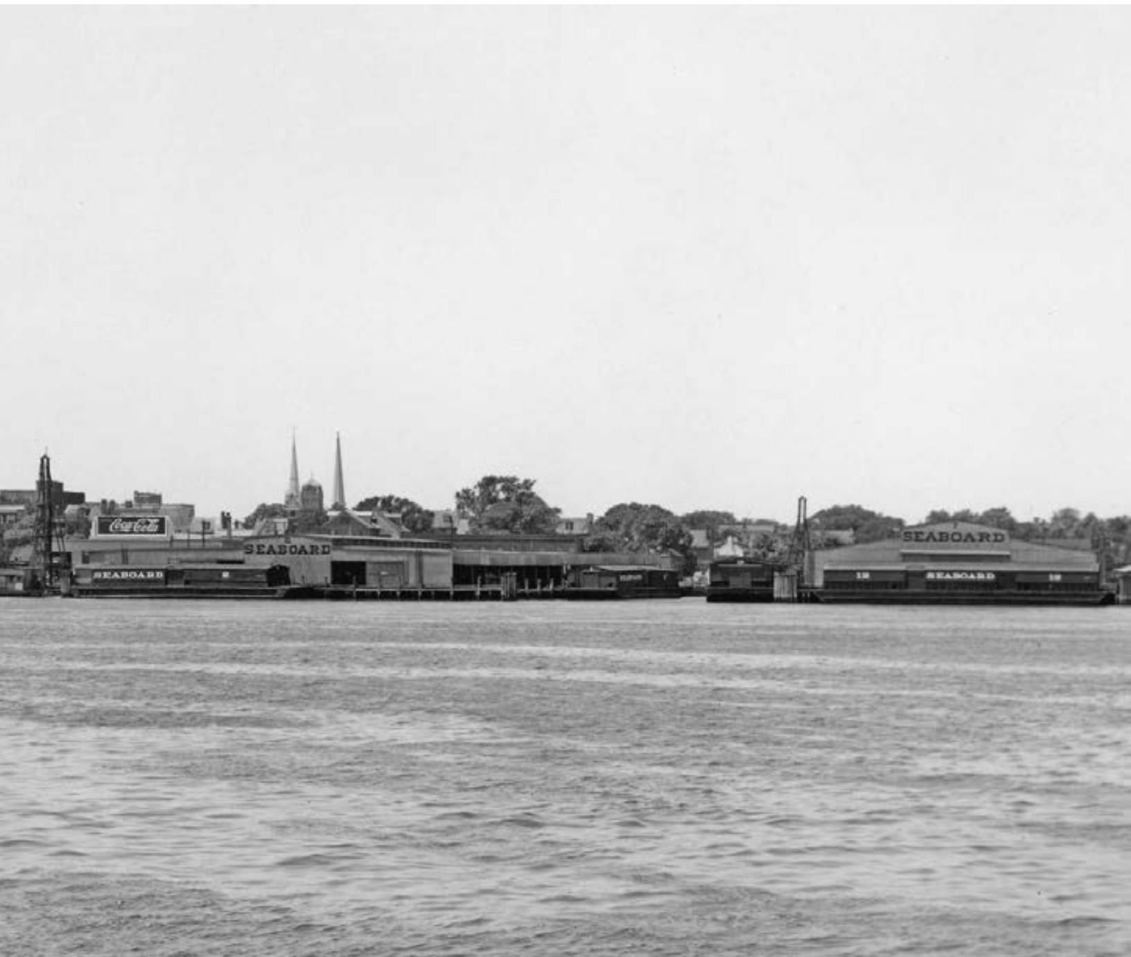
Below: Seaboard once had this extensive warehouse complex at its Portsmouth waterfront terminal, along the west bank of the Elizabeth River. A number of the railroad's lighters (covered barges) are visible in front of and between the warehouses; they were used to transfer freight to the railroad's Norfolk freight station. —SAL photo, Robert Wayne Johnson collection
