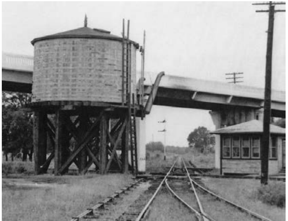
Above: This photo was taken on the ACL Florida Southern Route looking railroad north toward High Springs about 1942, with BX Tower, the water tank and its two spouts, and Highway 441 in view. Visible in the foreground are the points of the only switch controlled by the interlocking plant, the short connector from the Florida Southern Route. The J&SW line between Jacksonville and Wilcox can be seen crossing in front of BX Tower and the SAL line is crossing beyond BX. — F.W. Thomas photo, L.A. Bailey collection
