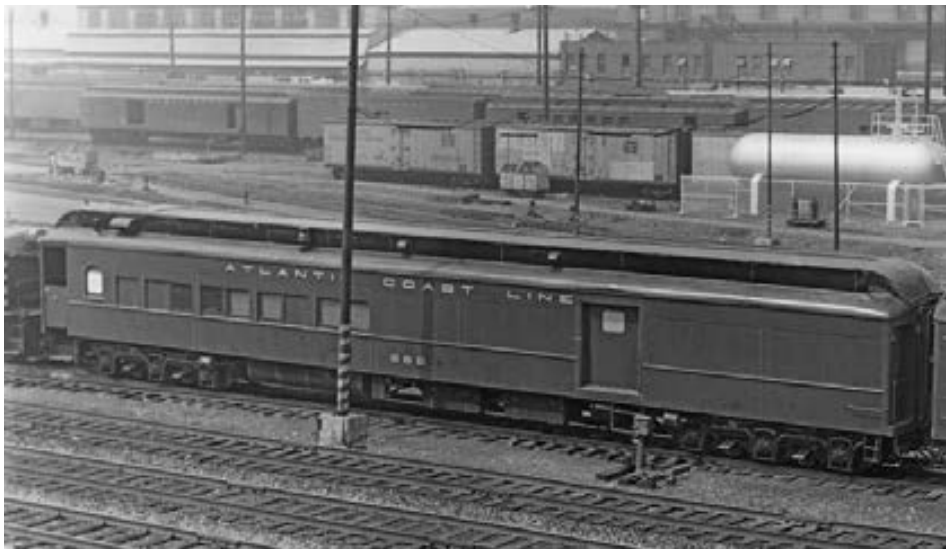
Above: Baggage-coach 666 was assigned to Atomic Energy Commission service between the Savannah River Plant near Augusta and Rocky Flats, Colo., carrying material to manufacture nuclear weapons. The car's interior was rebuilt to accommodate lead-lined containers and dormitory space for armed guards. This circa mid-1960s photo shows it in Chicago. — Jay Williams collection
