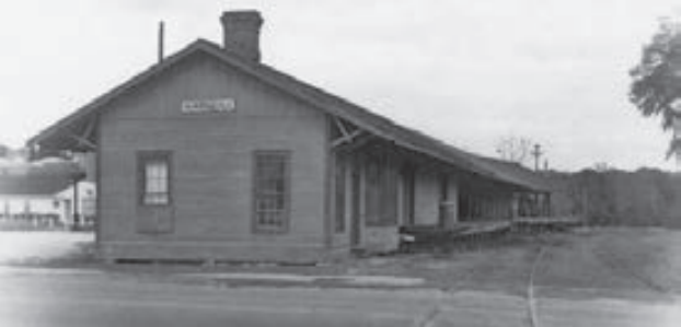
Above: This 1970 photo is the former SAL Alachua depot on the Newberry line, now under SCL ownership. It was just one short block north of the ACL depot on the Newberry line. This wood frame structure had a lengthened, open freight platform, giving the impression that agricultural freight business had been very good in the earlier years. —Ken Murdock collection
