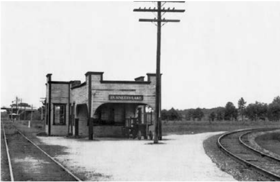
Left: The Burnett's Lake depot was a very unusual design that didn't following any of ACL's standard depot designs. It appears to be an attempt to create a wood version of the Spanish-styled stucco structures popular in Florida in the early 1920s. It was very primitive, never having boarding platforms or a paved access road. This circa-1942 photo was taken looking towards High Springs on the Florida Southern route with Gainesville to the photographer's back. The home signal, BX Tower, and the U.S. Highway 441 overpass can be seen in the distance. The long connector or north leg of wye from the Florida Southern Route to the J&SW is on the right. — F.W. Thomas (BX Tower operator) photo, L.A. Bailey collection
