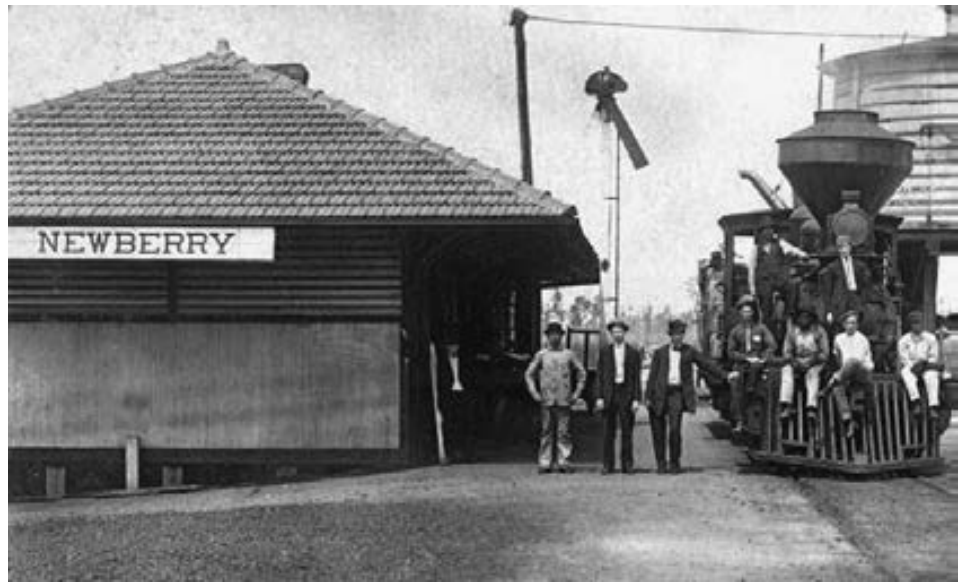
After purchasing the J&SW, ACL built this new depot at Newberry in 1908. The station was quite an elaborate facility with special wood siding and a tile roof. Note the lower quadrant order board and the water tank on the right. Observing the sloping terrain at the base of the depot, it appears to have been built at a different location than the first. Frequently, the old depot was saved and used as the freight depot. — Florida Archives photo pr7637
