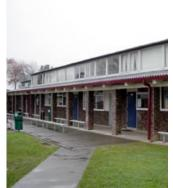
Hackshaw designed a series of buildings for this large site. The first, dating from 1962, was a compact two-storey classroom block. In a cost-cutting pattern Hackshaw would often reuse, the building avoids internal circulation spaces - the upstairs classrooms are accessed from two covered but external staircases.
