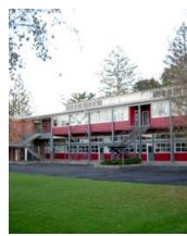
Running parallel to West Tamaki Road, this project boldly added a second floor to a block of existing classrooms. Wedged between a two-storey classroom block and the school hall, and overlooking a large, grassy courtyard, the elevated row of classrooms are supported by an exposed, steel skeleton.
