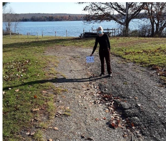
Roads and driveways built to access new development can deliver large quantities of sediment and attached P if not built correctly or maintained properly. (Photo Credit: CLA)
