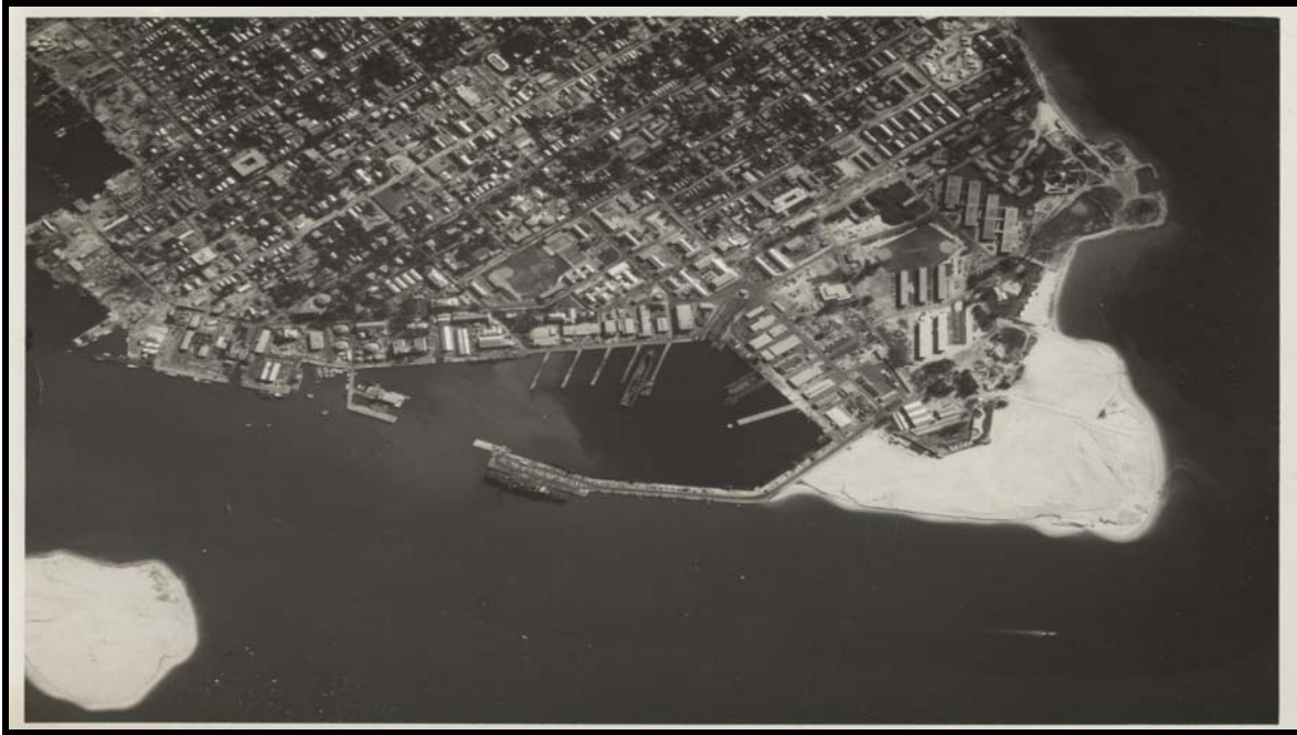
FIGURE 3.A.10. FILLING PROGRESSING OFFSHORE AROUND FT. TAYLOR AND ON TANK ISLAND IN THE 1950S (FARALDO COLLECTION).
