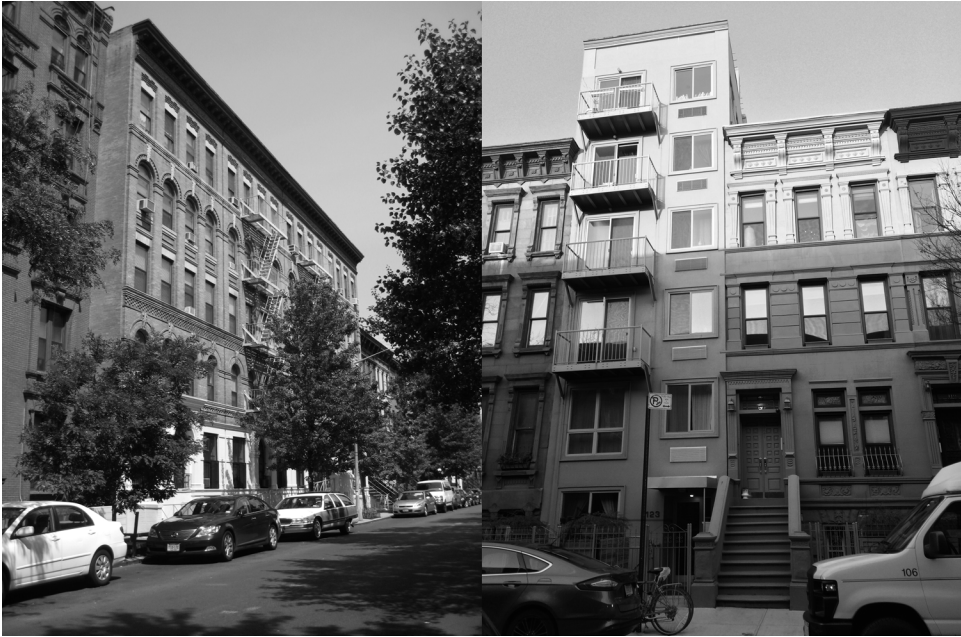
Figure 5. By the late twentieth century, new development in Harlem typically retained, repaired, or sensitively replaced the neighborhood's built fabric, but the residents of such housing were increasingly affluent. Pictured here are two examples, both on West 131st Street. Shown on the left is West One Three One Plaza, a middle-income condominium building developed by a Harlem-based community development corporation and completed in 1993. Harlem Sol, a privately developed condominium building, is shown on the right. Involving the restoration of a historic brownstone and contextual new construction, the structure was completed in 2011. Photographs by Brian D. Goldstein. Courtesy Brian D. Goldstein.
