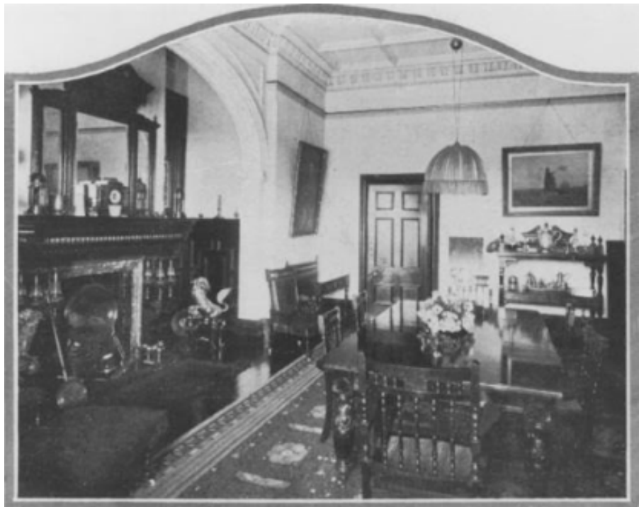
Restored Boardroom at Ross Roy
