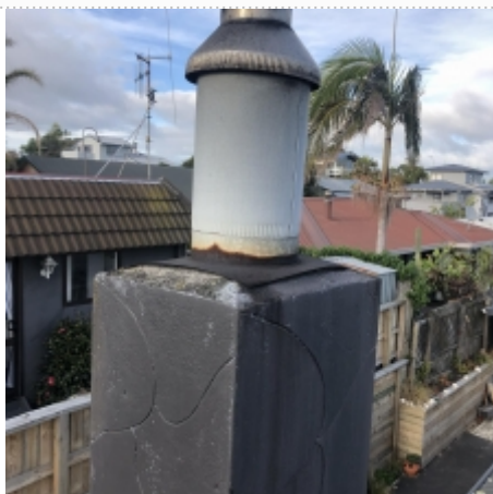
Pic 1: Chimney cowling rusted
