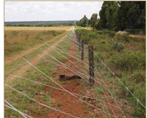
The new short-post fence design
