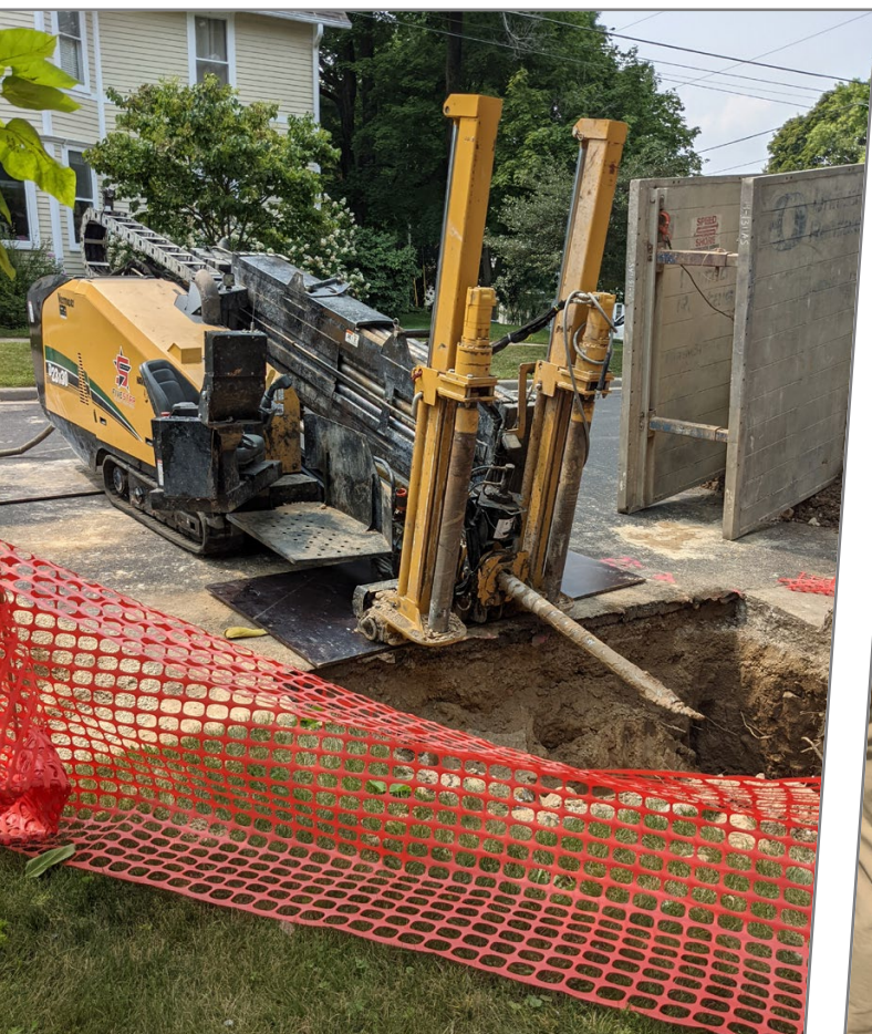
The bulk of the expense of replacing lead service lines comes from the costs of heavy machinery and labor, rather than from the cost of the replacement piping, regardless of what piping material is used. Lead service line replacement in progress in Stoughton, Wisconsin. Images by Casey Sweeney, courtesy of the Wisconsin Department of Natural Resources.
